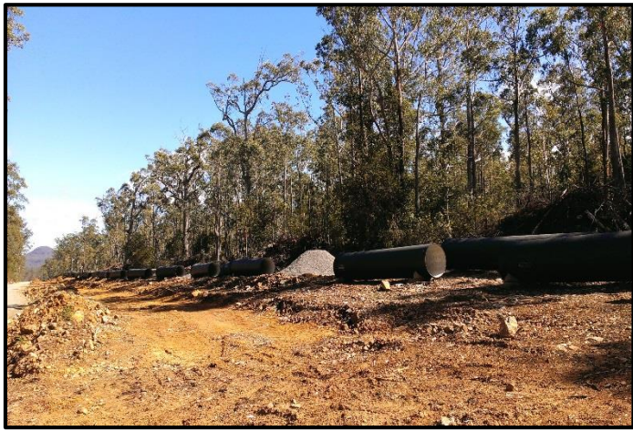
Photo: Large pipe work 1m diameter, laid out in the pipeline corridor before being connected and buried.
