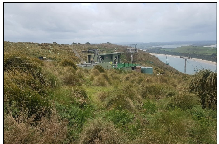
Photos 6 & 7: Before and after photos showing the Gorse control progress around the chairlift station within 4 years.
