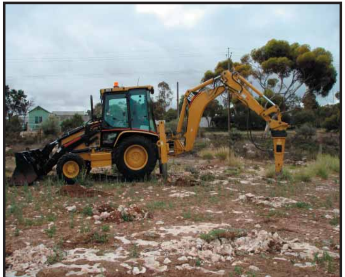
Above: Rock Breaker working on holes in limestone
